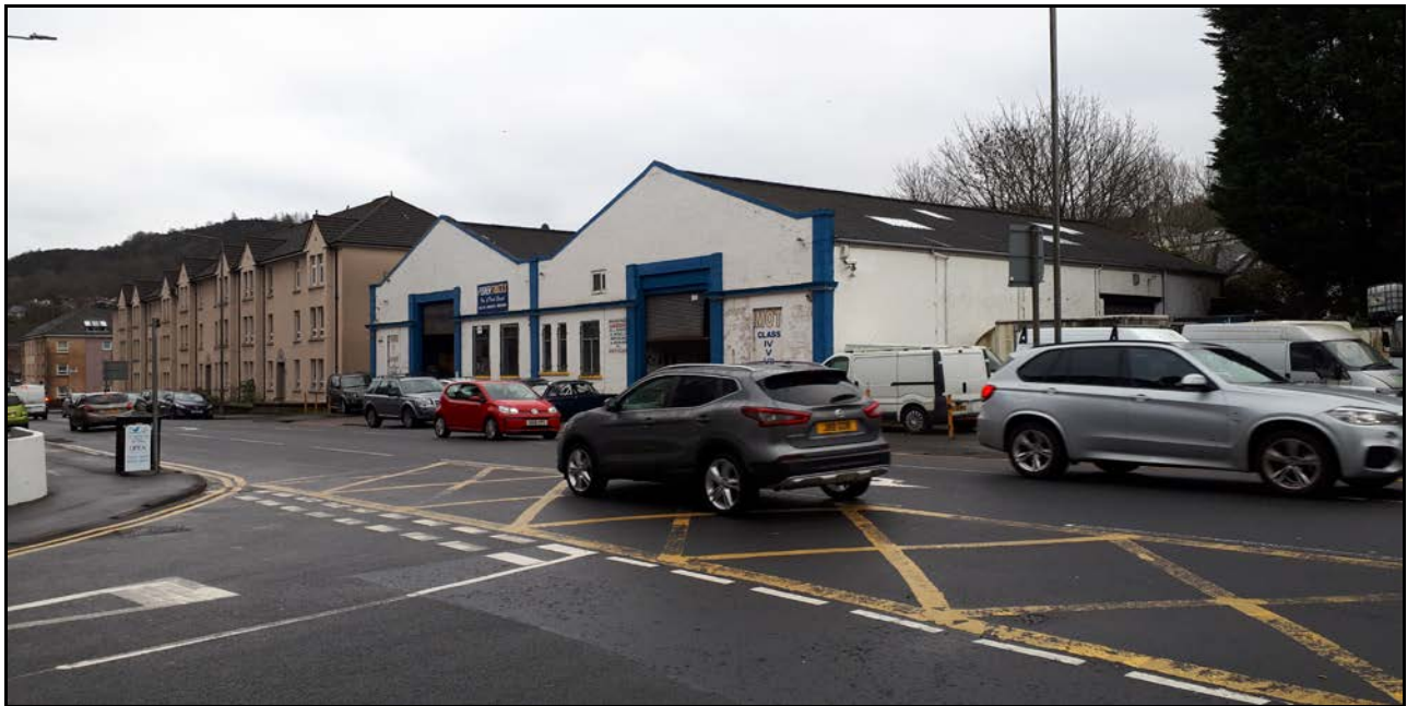
Looking south-eastwards at the junction with Tarbet Street
