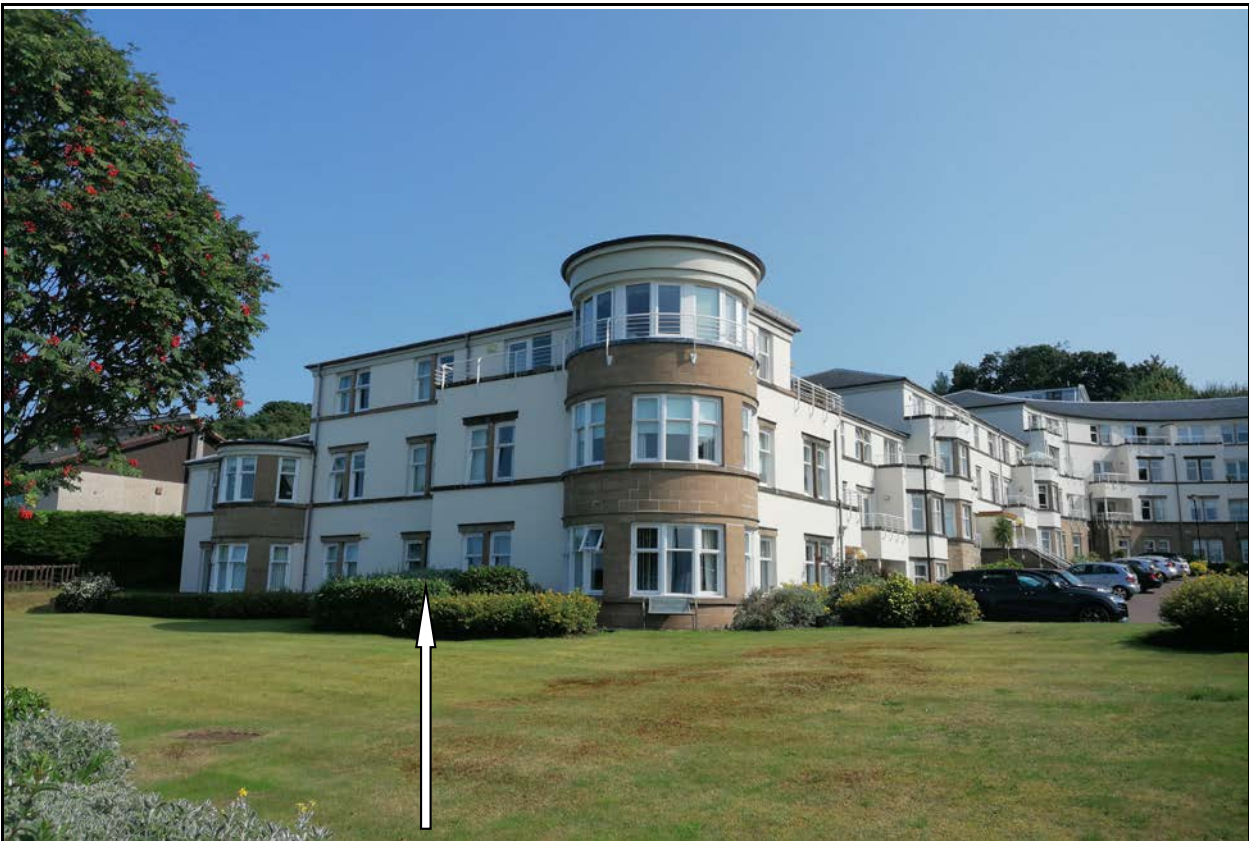
View of the building from Cloch Road. Window in question is seen as partially obscured from this angle.
